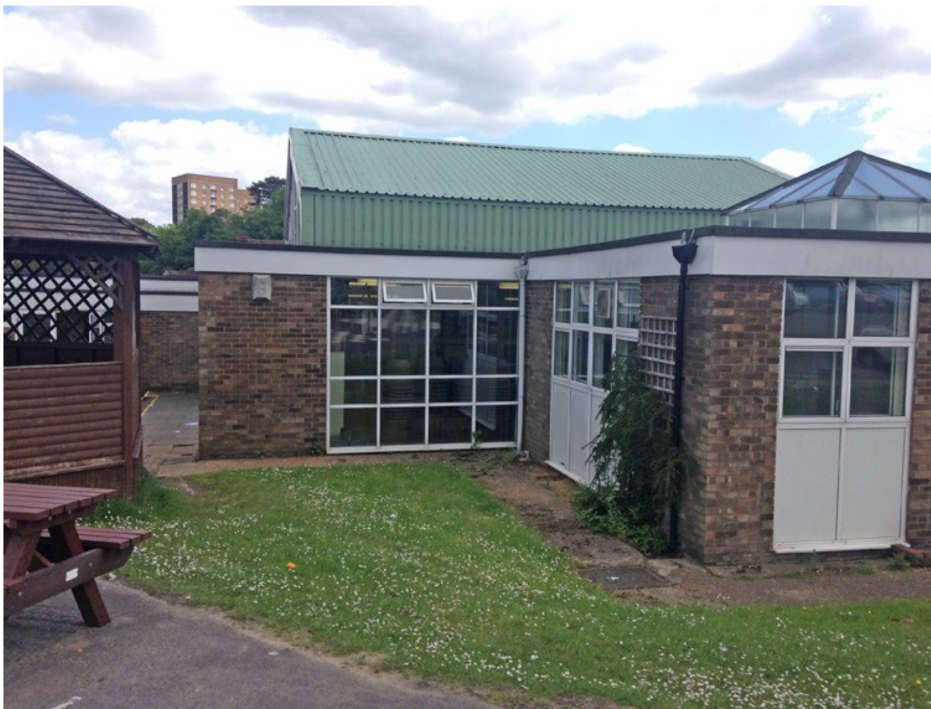
Figure 5 : View of the location of the proposed kitchen extension facing south east
